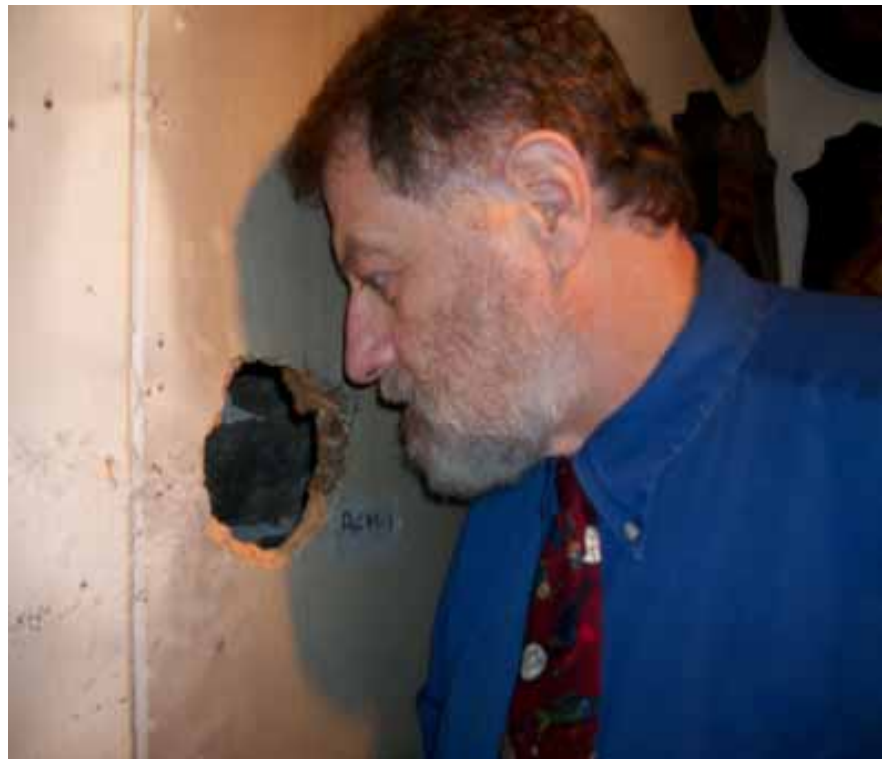
Past President Gary Green confirms the lack of insulation in the Club walls.
